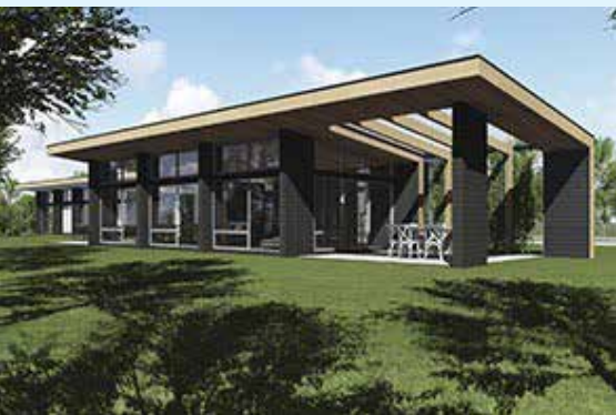
Ngunguru Road, Passive Solar House
